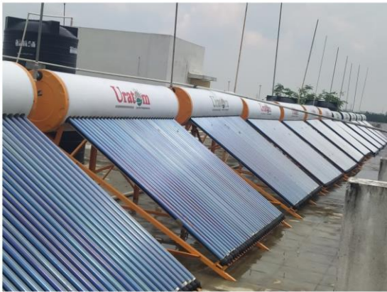
Photo 2 Solar Water Heater
